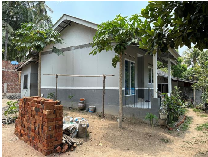
Fig. 2: A RIKO house with a low brick wall and fibre board wall infills above ( photo: lead author, 2023 ).
